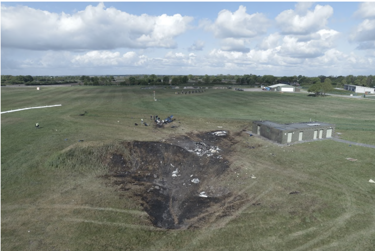
Fig. 10: Accident site, view direction about 260°
