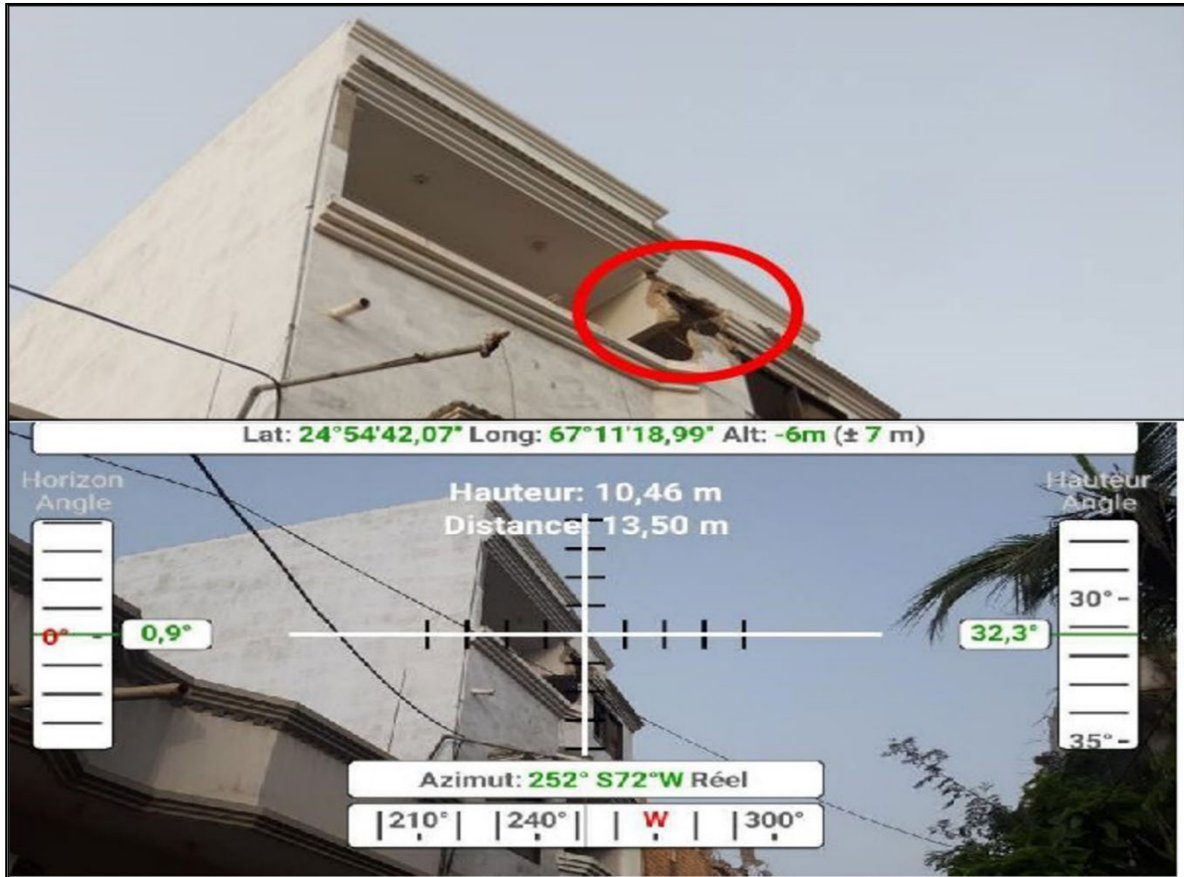
Figure 23 – Impact Point at Height 10.50 m and 46 m Distance from East End of Street
