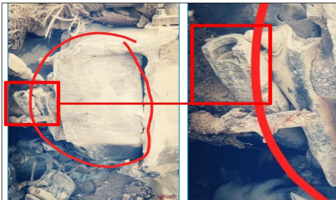
Figure 67 – Heavy Rubbing on End Fitting Installed on Hose
