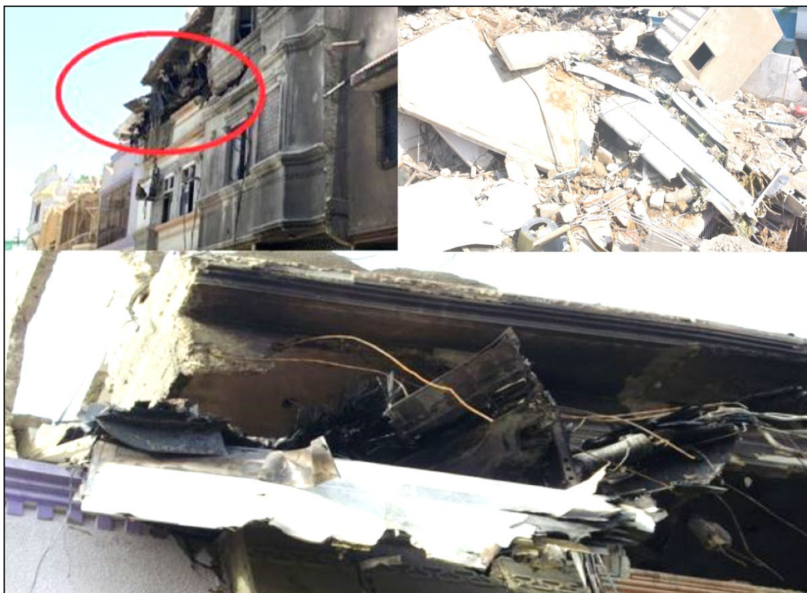
Figure 35 – Left Wing at Rooftop
