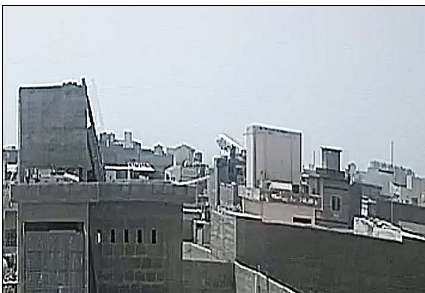
Figure 19 – CCTV Footage before Impact
