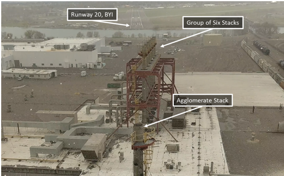
Figure 9. Image of the Gem State Processing plant roof top. The agglomerate stack and the group of six stacks are in view. Photo courtesy of the Hayburn Police Department.
