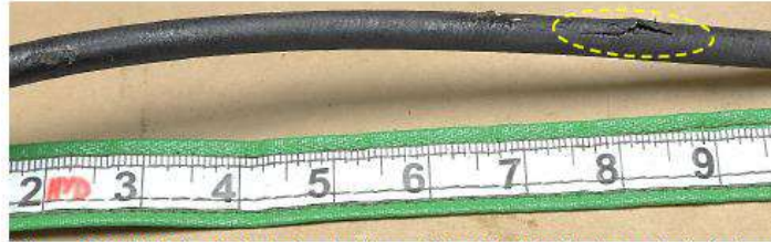
Figure 20: R/H MLG downlock actuator extend hose. Yellow-dashed circle indicates a tear in the hose abrasion sleeve
