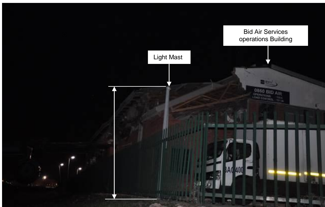
Figure 6 Light Mast damaged in the accident
