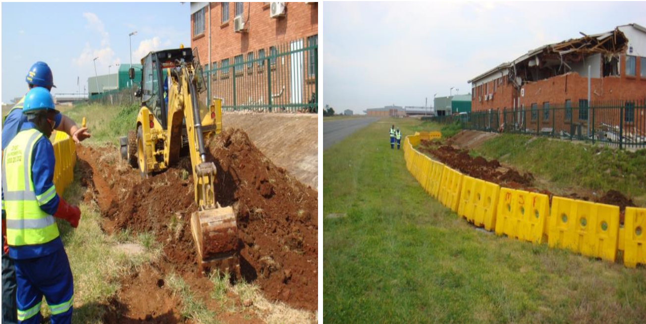
Figure 11 and 12 Remediation of the fuel spillage area
