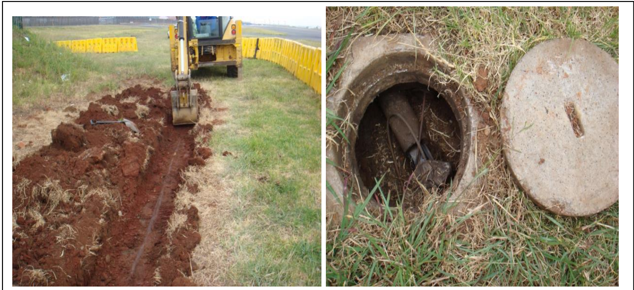
Figure 13 Electrical and Fibre Optic cables detected underground
